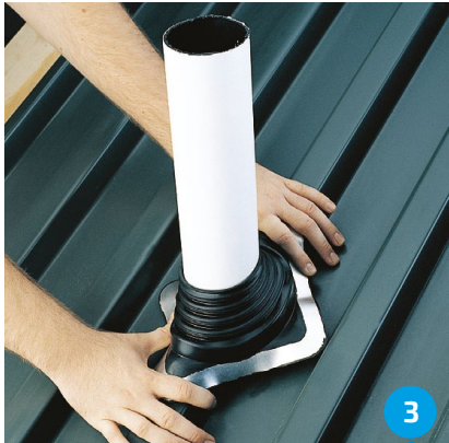
3 Press Master Flash® down, bending it to conform to roof profile or roof irregularities. A blunt tool will help press the flashing into tight roof angles.
