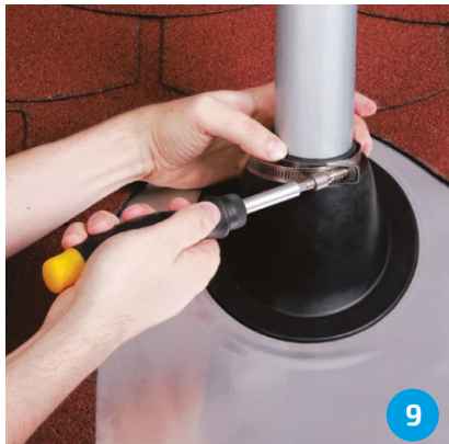
9 Apply a stainless steel band to assure tight fitting of the flashing against the pipe.
