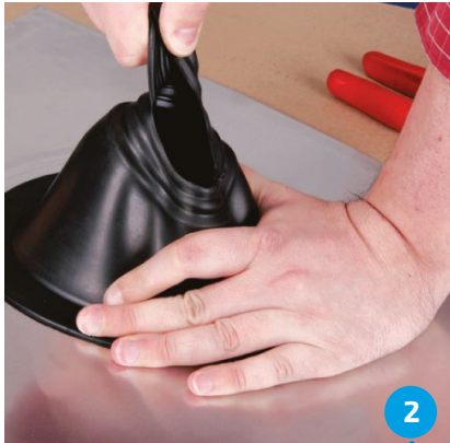
2 Finish the diameter by adjusting the flashing by hand.
