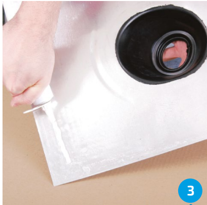
3 Apply sealant on the bottom side of the metal base.
