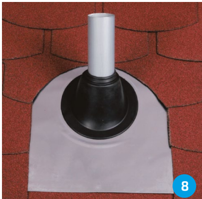
8 Finish the installation of tiles.
