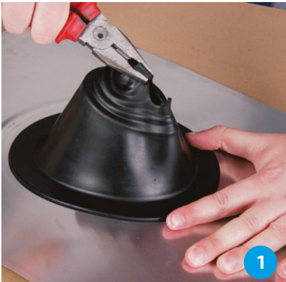
1 Use pliers to pull the tab for the correct pipe size.
