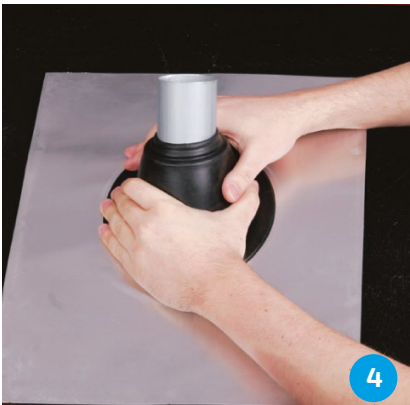
4 Slide the flashing down the pipe.
