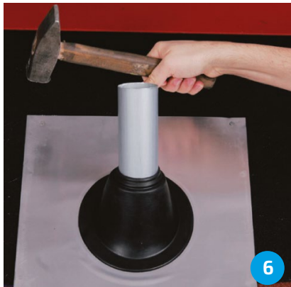
6 Fasten the metal base using nails and a hammer.
