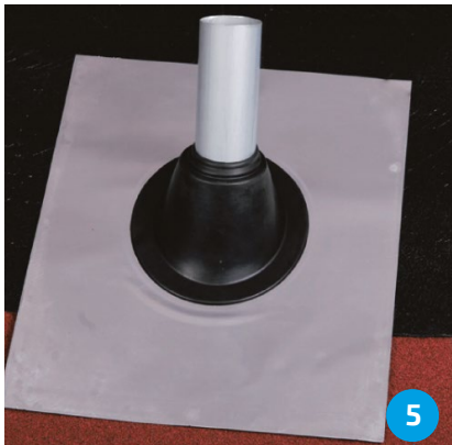
5 Cut shingles to fit to the top of the flashing allowing the bottom of the flashing metal base to set on top of tiles.
