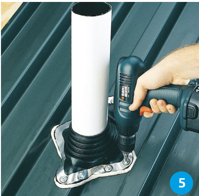
5 Use fasteners to complete sealing. For installation, fastener spacing may not exceed 1.5" (38 mm).
