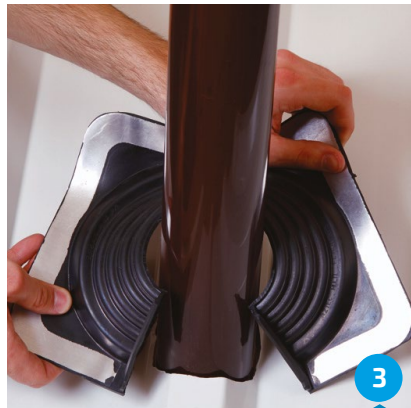
3 Wrap Master Flash® Multi around the pipe.
