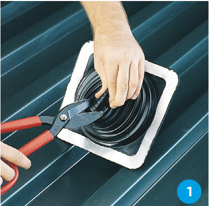
1 Choose an appropriate Master Flash® with opening at least from 20% to 30% smaller than pipe diameter. If necessary trim opening to 20% smaller than the pipe diameter.
